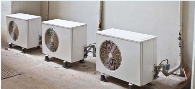
Figure 6.6 : Installation of ODU
