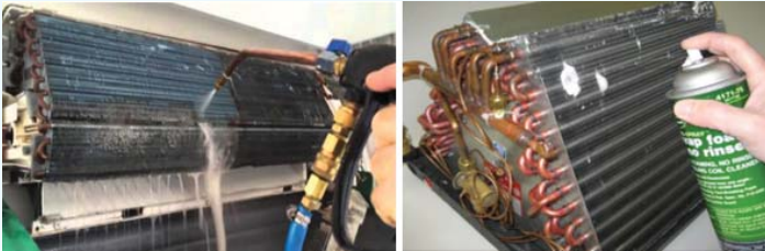
Figure 8.3 : Cleaning of condenser and evaporator coils
