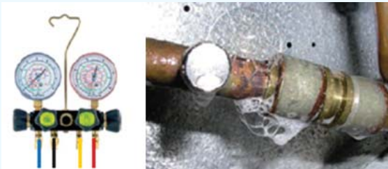
Figure 8.7 : Leak and Pressure Testing
